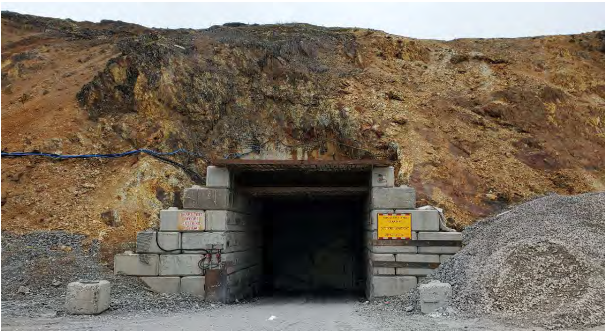
Figure 3.7-9. West Zone Portal (Photo July 2020).
