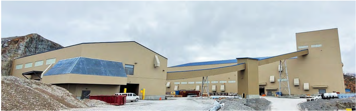
Figure 3.7-8. VOK Portal Building, Tower and Conveyor Gallery (Photo July 2020).
