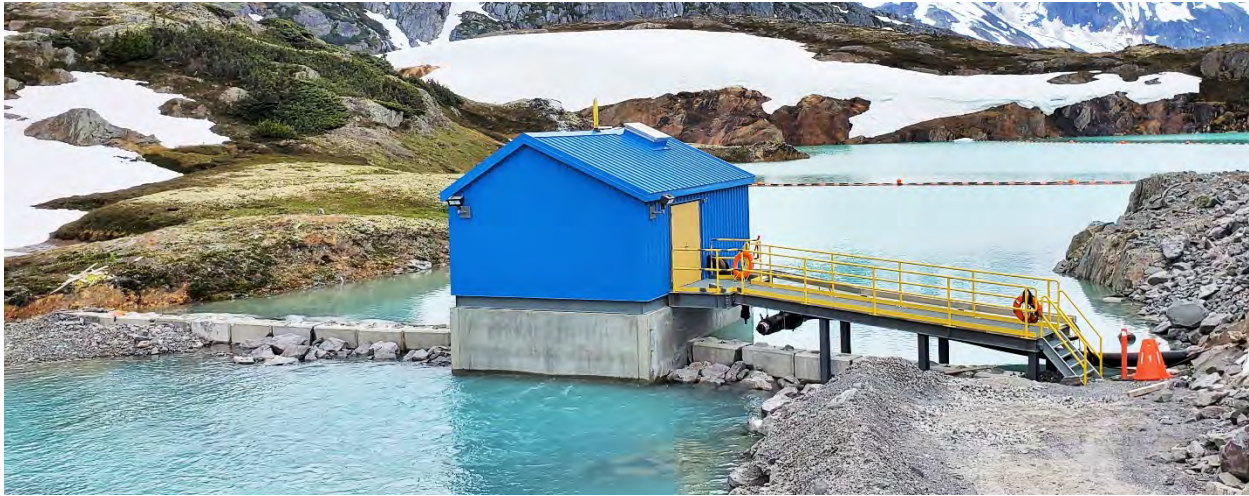
Figure 3.7-18. WRTSF Outlet Weir (Photo July 2020).
