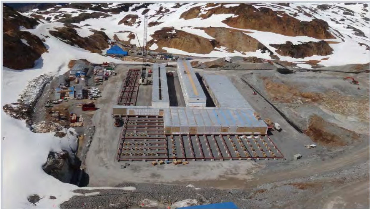
Figure 3.7-6. Modular Phase 2 Camp Complex During Construction in 2016.
