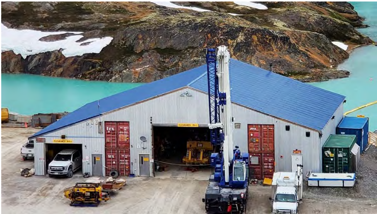
Figure 3.7-11. Surface Heavy Shop (Photo July 2020).
