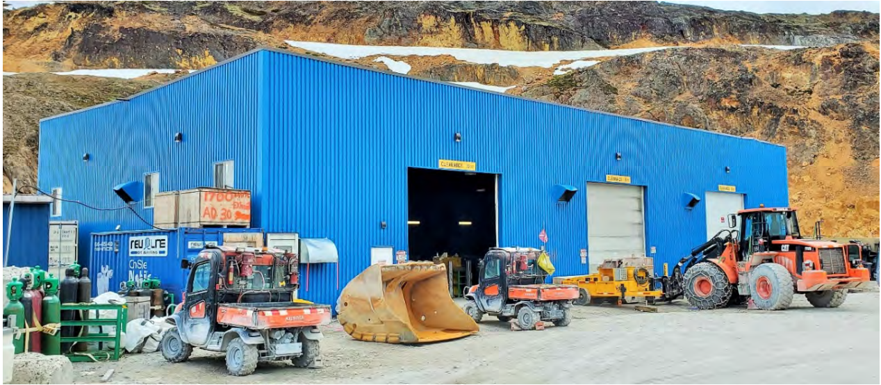
Figure 3.7-12. West Zone Heavy Shop (Photo July 2020).
