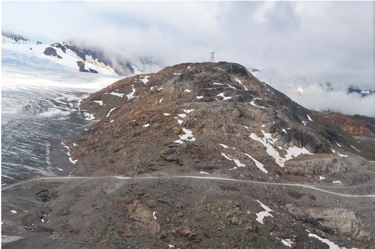
Figure 3.3-3. Transmission Line Towers in Northernmost Bedrock and Ice Section (Photo July 2018).
