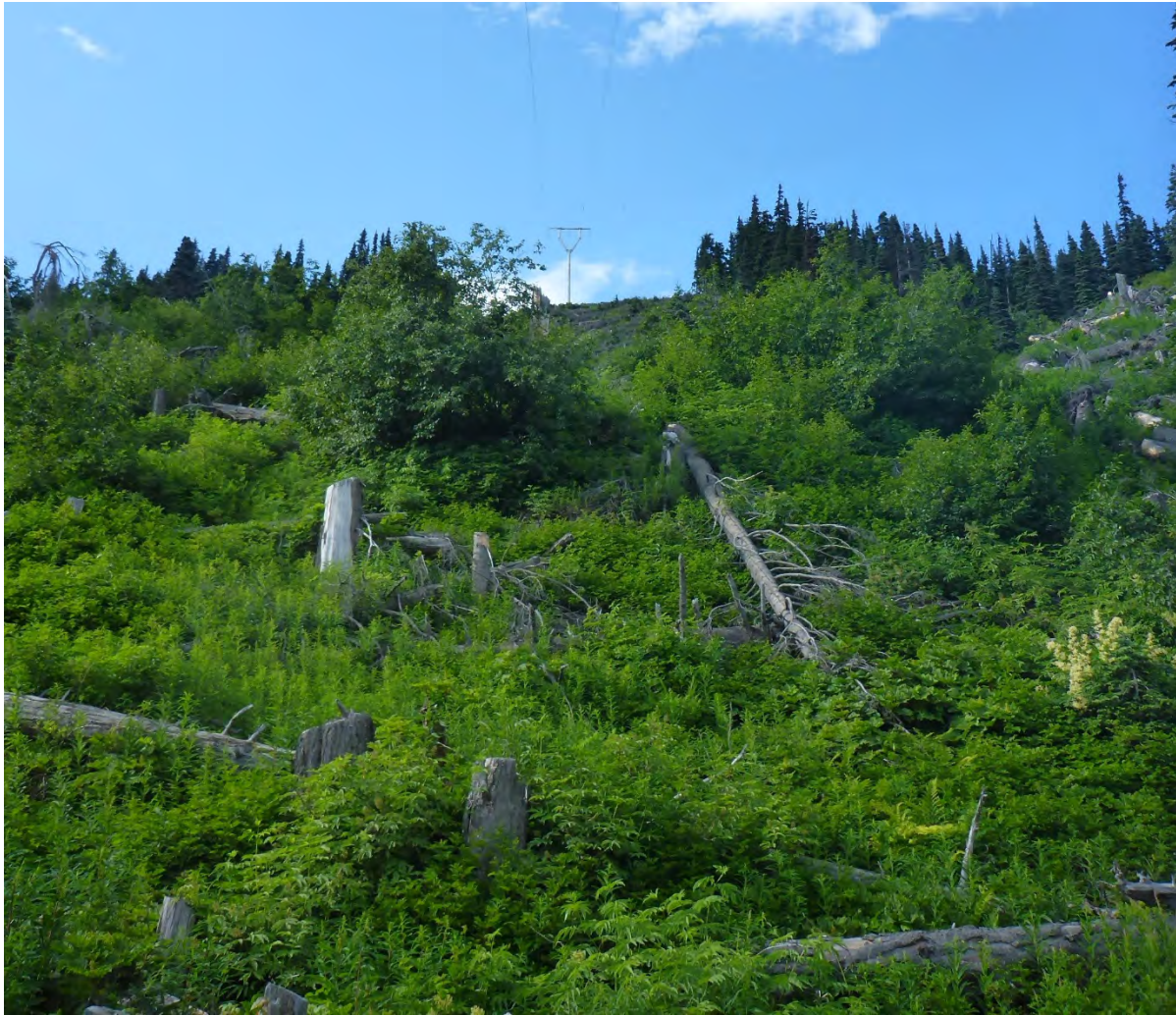
Figure 3.3-10. Transmission Line Natural Vegetation Cover Following Clearing (Photo July 2020).
