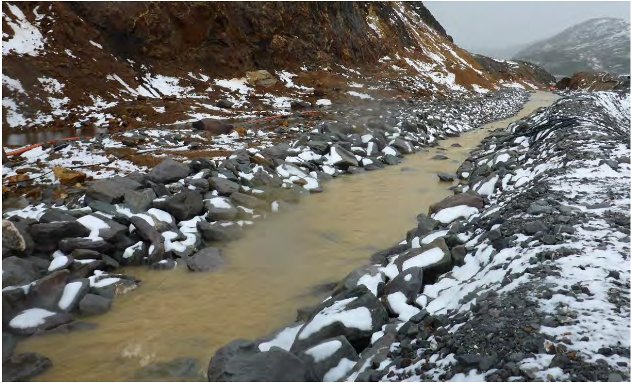
Figure 3.7-16. Camp Creek Diversion Channel (Photo July 2020).
