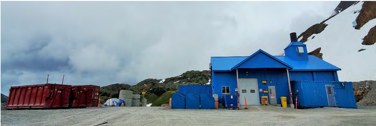
Figure 3.7-14. Incinerator and Waste Sorting Facility (Photo July 2020).
