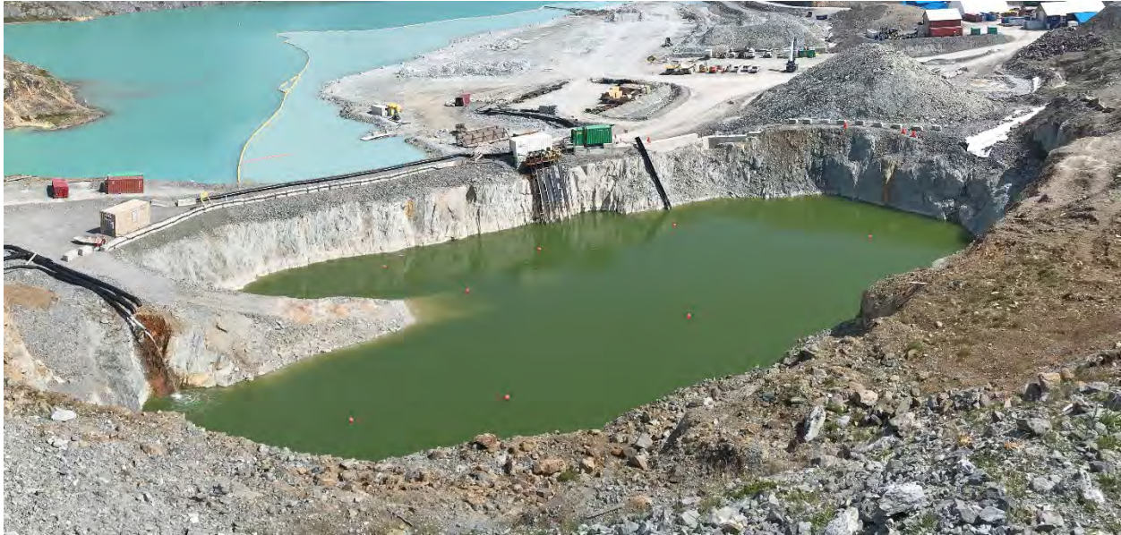
Figure 3.7-17. Contact Water Pond.
