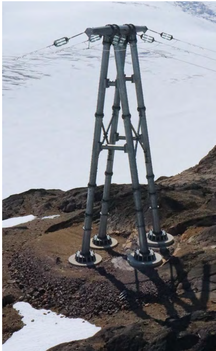
Figure 3.3-4. Transmission Line Tower, Northernmost Transmission Line Section (Photo July 2020).
