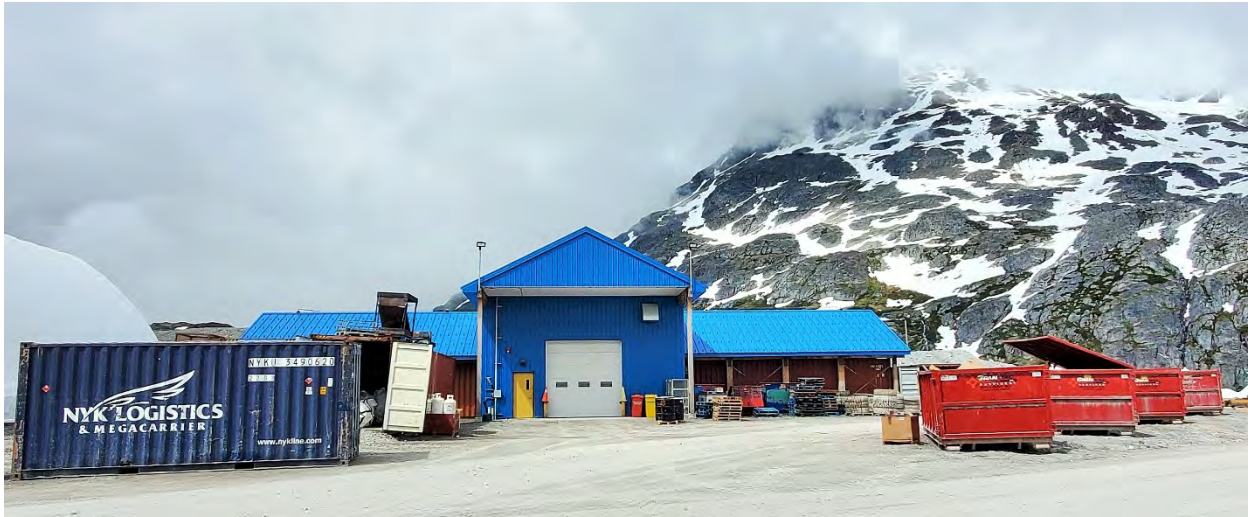
Figure 3.7-13. Primary Waste Sorting and Staging Facility (Photo July 2020).
