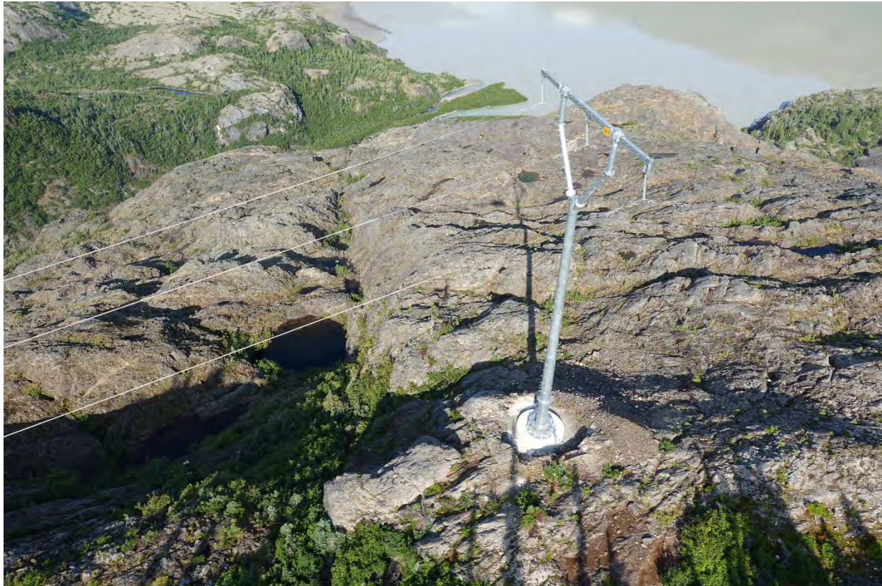
Figure 3.2-3. Transmission Tower on Bedrock in M-243 Vegetated Section (Photo August 2019).
