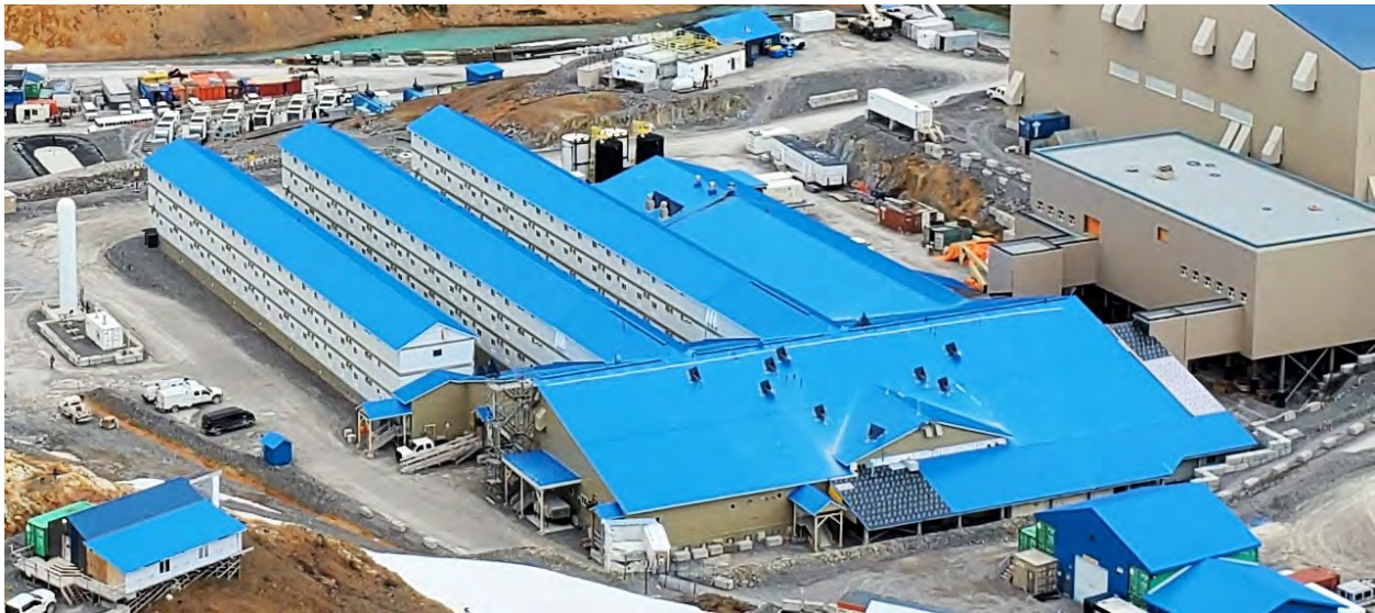
Figure 3.7-10. Phase 2 Camp Complex (Photo July 2020).
