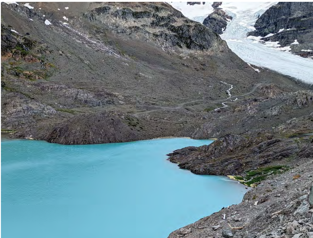
Figure 2.2-3. Initial Mine Access Road Section North of km 72 NPAG Quarry Constructed in 2015
