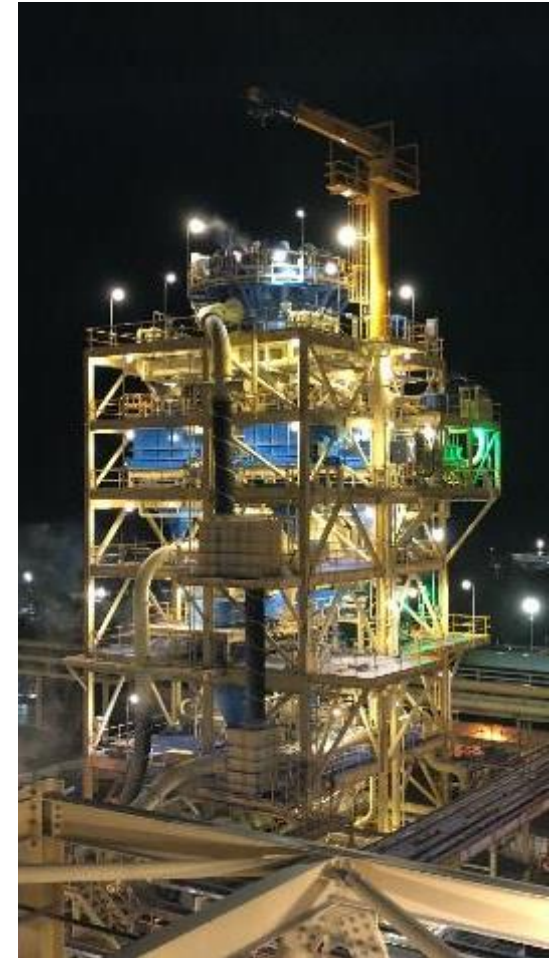
Coarse ore flotation plant, Cadia
