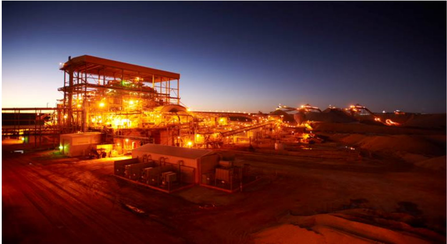
Telfer Processing Plant
