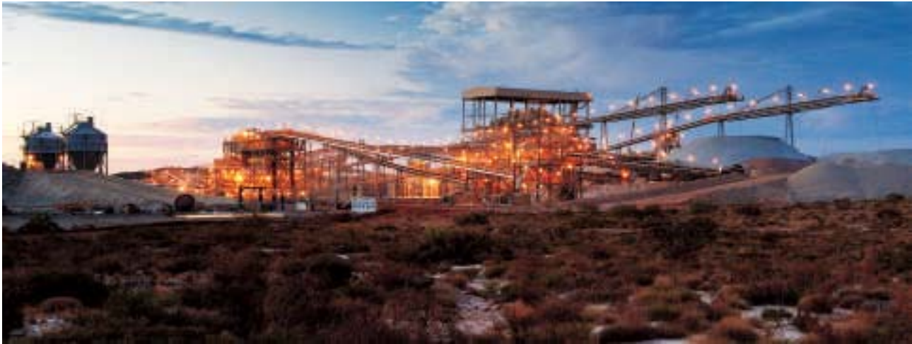
The newly constructed Telfer processing facility.
