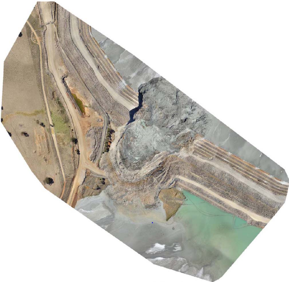
Aerial view of failure zone
